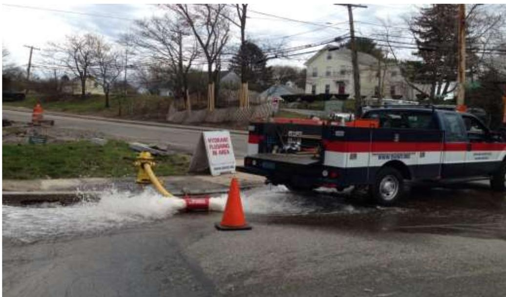
*Water Main Flushing to remove sediments from pipes*
