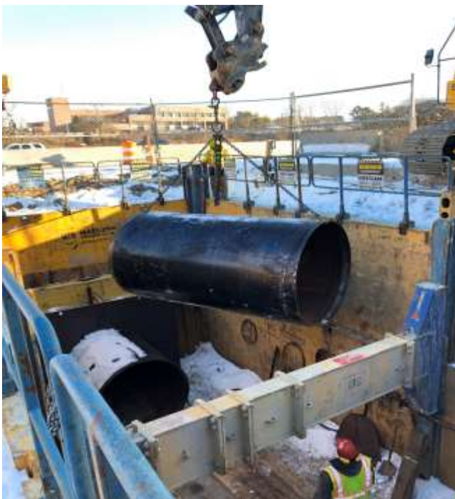
Installation of pipe underneath Route 128 at the East Street Rotary joint project with MWRA
