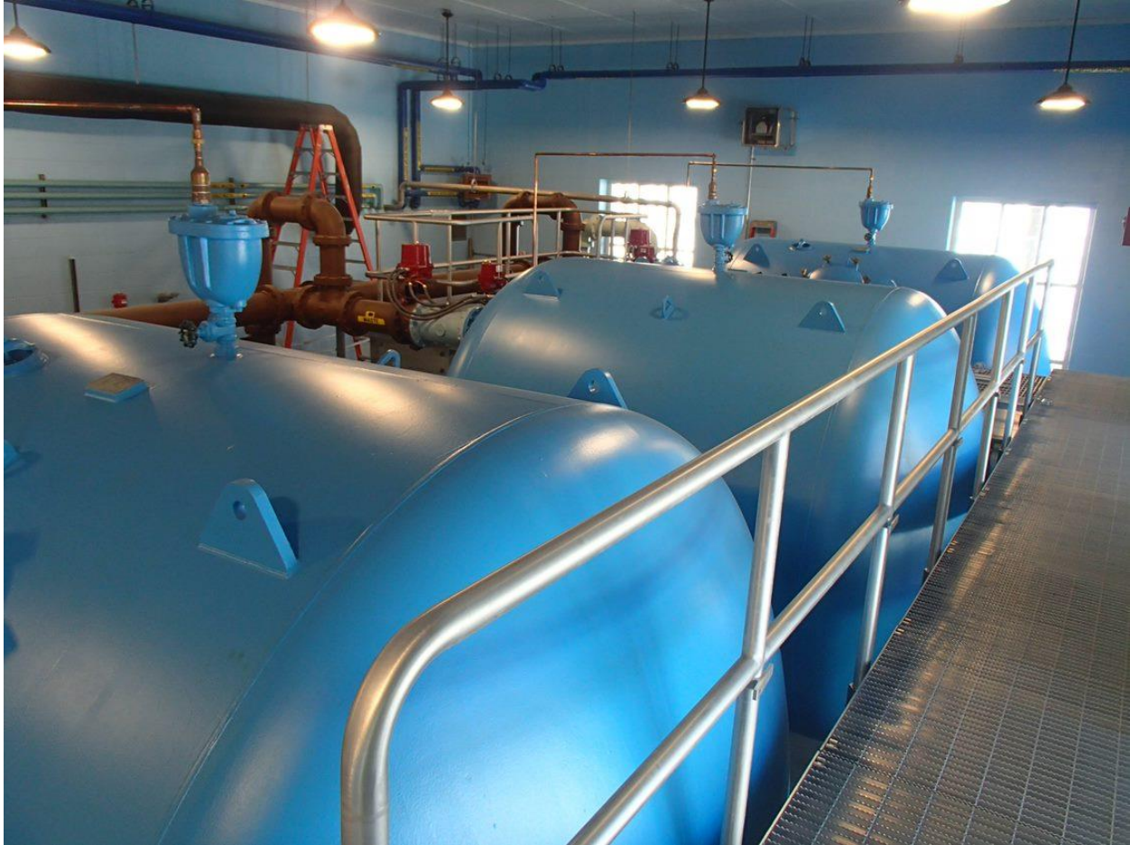
DWWD New Water Filters Bridge Street Treatment Plant Modernization project
