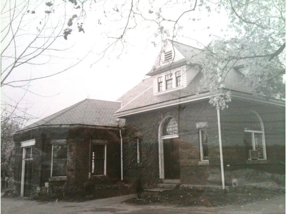
Bridge Street Treatment Plant and Pump Station
