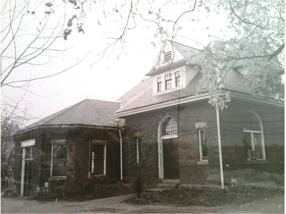
Bridge Street Treatment Plant and Pump Station
