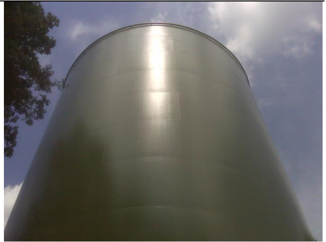
FOX HILL WATER TANK
