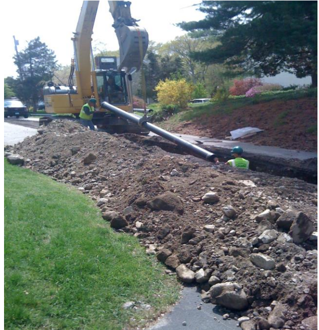
Beechnut Road Water Main Installation
