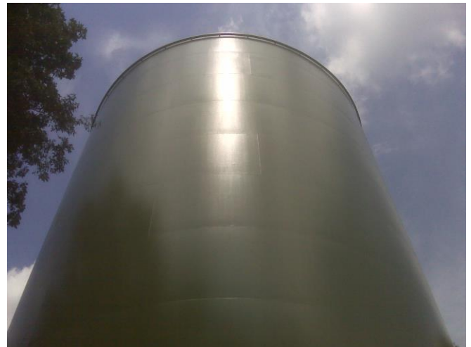
FOX HILL WATER TANK
