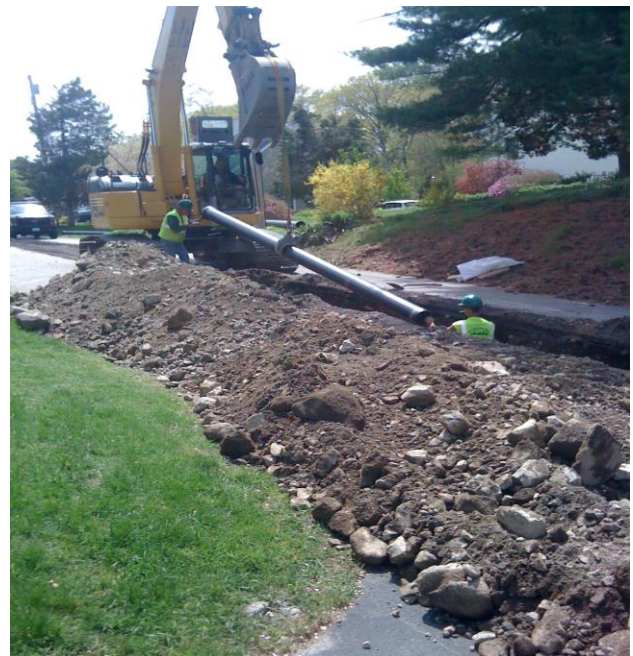
Beechnut Road Water Main Installation
