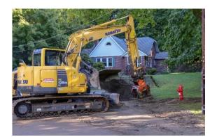
An excavator is making the finishing touches around a newly installed fire hydrant.
