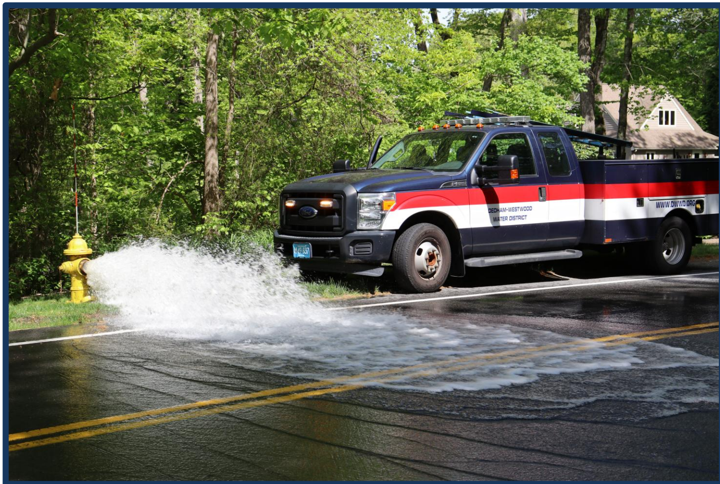
Image Above: Water main flushing via fire hydrants on Summer Street in Westwood.
